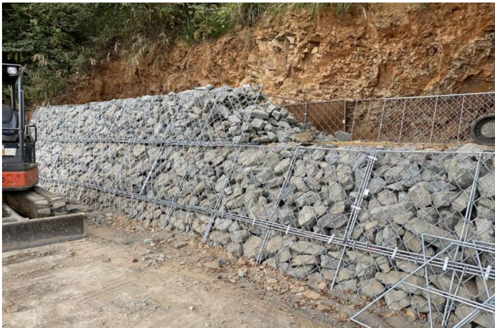
Figure 6.11 Gabion Check Dam
