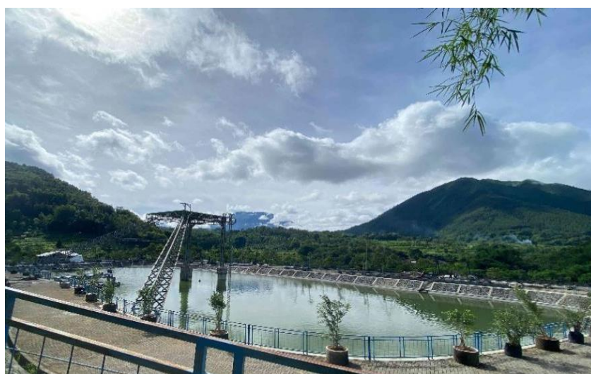
Figure 6.23 Application of Water Reservoir
